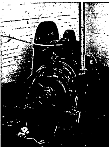
Electric motor for traction elevator.
