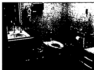
Resident toilet room in 1978 addition; note lack of rear grab bar.
