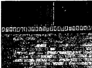
Mortar joints at sill deteriorating.
