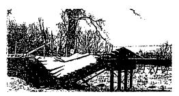
An example from Tripp County is pictured, but it is not the only case. In the past two years alone, six county bridges had to be completely replaced because of damage from illegally overweight trucks:
