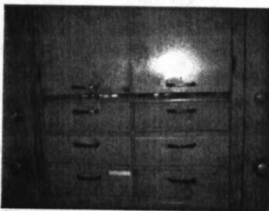
Exhaust air is drawn through gap between upper and lower portions of storage unit.
