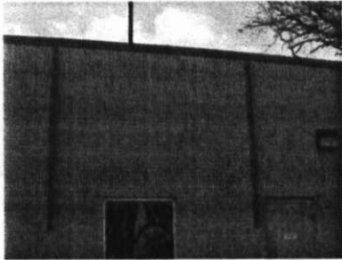
Angles used to secure tie rods through building.
