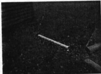
Exposed PVC storm drainage piping near Gazebo.
