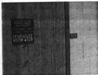
Non-compliant room and door sign.
