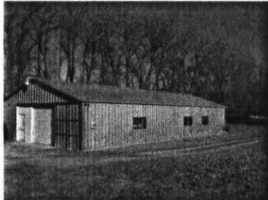
Metal storage building.
