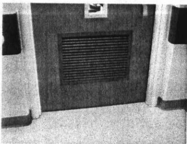
Louver on corridor door.
