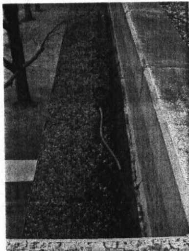
Built-up roof on sun shade.
