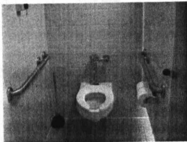
Toilet stall in original portion.
