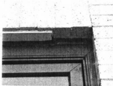
Lintel does not extend full width of opening.
