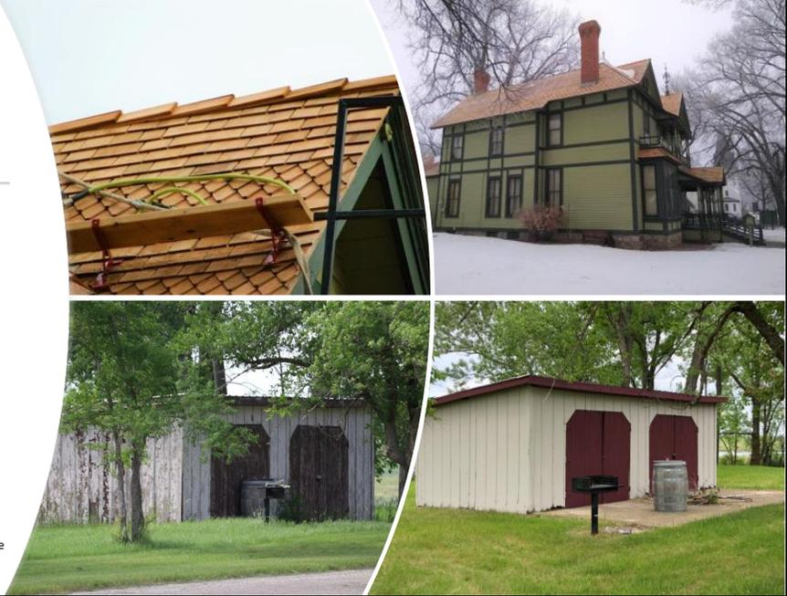
At the Former Governors' Mansion, cedar shingles and gutters appropriate to the time period of the Mansion were installed. In addition, the widow's walk was power washed and a new silicone roof coating applied.
