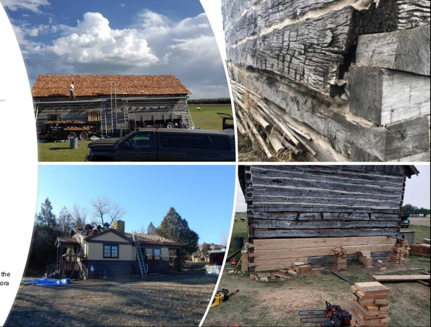
At Gingras Trading Post, the wall of the trading post was stabilized and the roof re-shingled.
