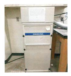
The current dust collector unit is undersized for the required duties and is reaching the end of its service period. A larger dust collector unit designed for continuous operation (as opposed to intermittent operation) is needed to handle the current scale of fossil preparation in the lab.
