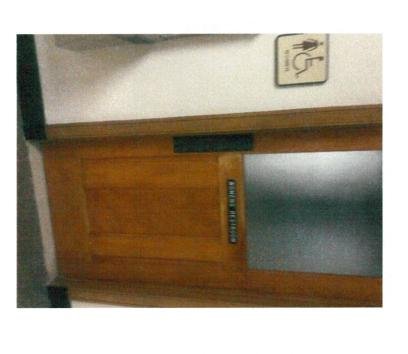
Accessible signage for Executive wing bathrooms should be removed, as they will not be ADA compliant based on door width alone
