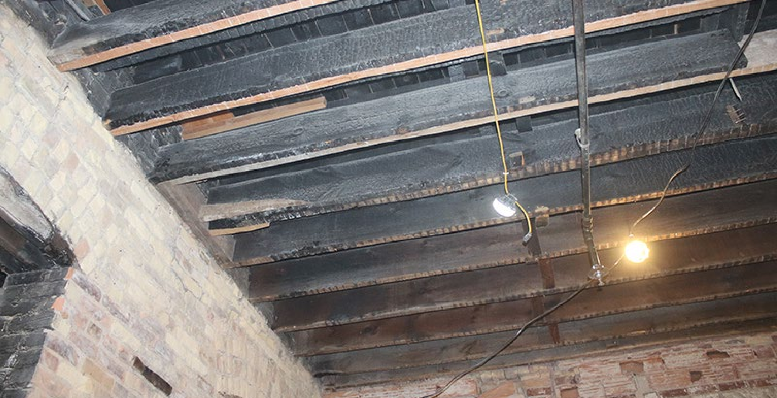
Evidence of 1925 fire can be seen in the rafters above first floor.
