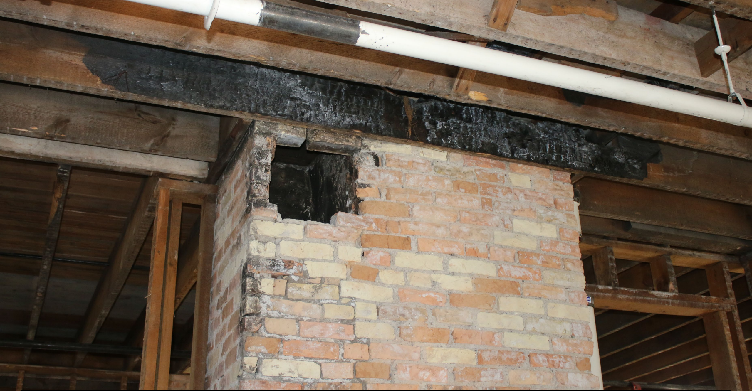
Evidence of a 1925 fire was revealed during the abatement process.
