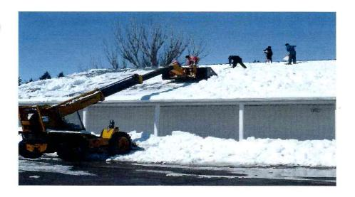
Community came out to help save the first two buildings by getting all the snow off the roof on the morning of April 6, 2023. The ceiling inside the second building was already leaking and was down about a foot inside. We knew rafters were broken by then.
