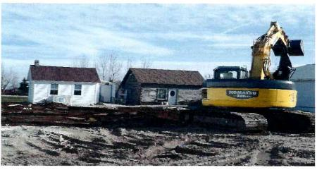
Prepping the site were building stood. We had to lose the concrete to the one room schoolhouse and log cabin and cut off some of the hallways to put the building back in the same spot.
