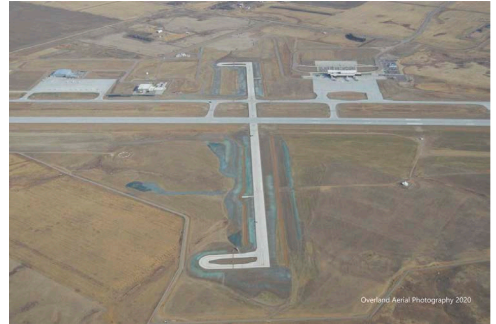
Williston Airport Crosswind Runway (2020)
