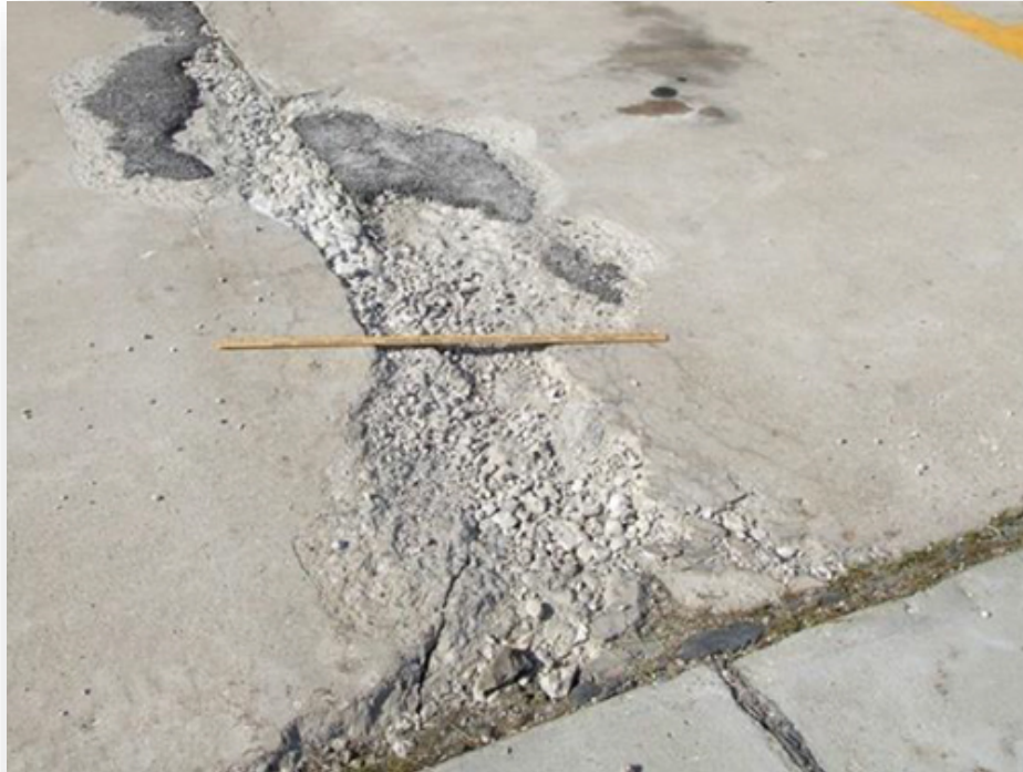
A yardstick for scale shows the amount of damage sustained by the concrete, as well as the potential for foreign object debris on UND's flight apron
