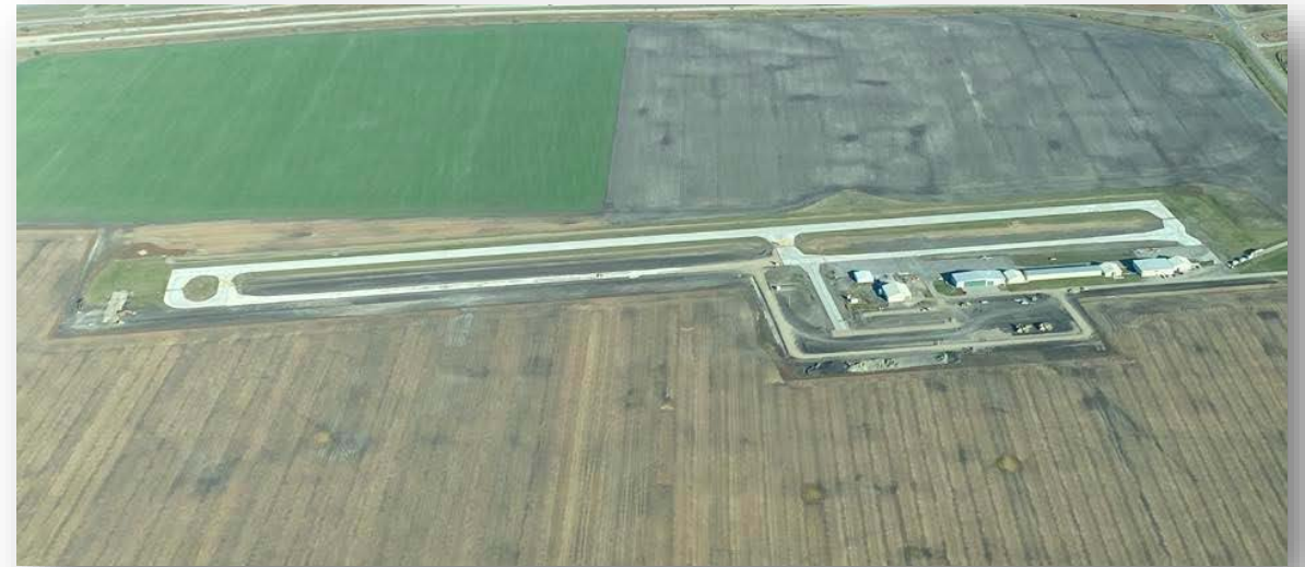
Hillsboro taxiway construction (2020)
