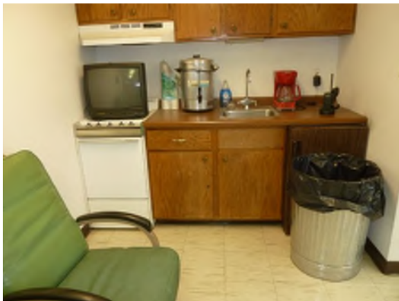
Kitchen appliances, casework, and fixtures not accessible
