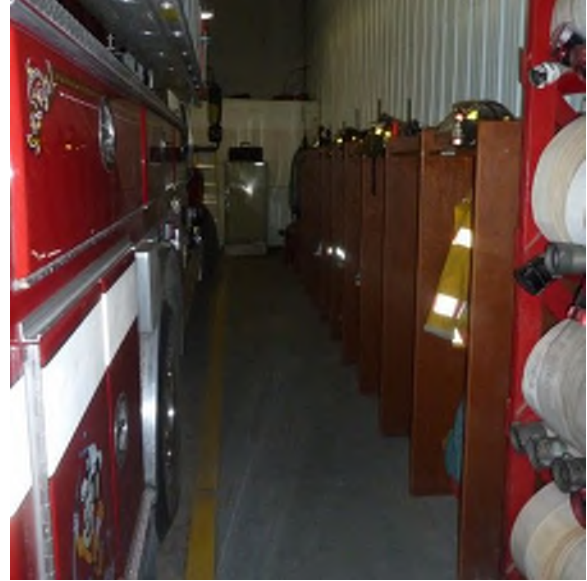
Turnout gear stored on bay walls too close to apparatus. Solid panels at gear lockers restrict evaporative drying of turnout gear
