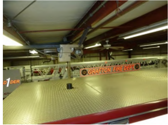
Roof and wall insulation compressed at each girt and purlin, rendering it less efficient at resisting each transfer
