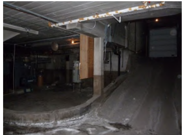
Access to fire boat in basement through door directly onto ramp
