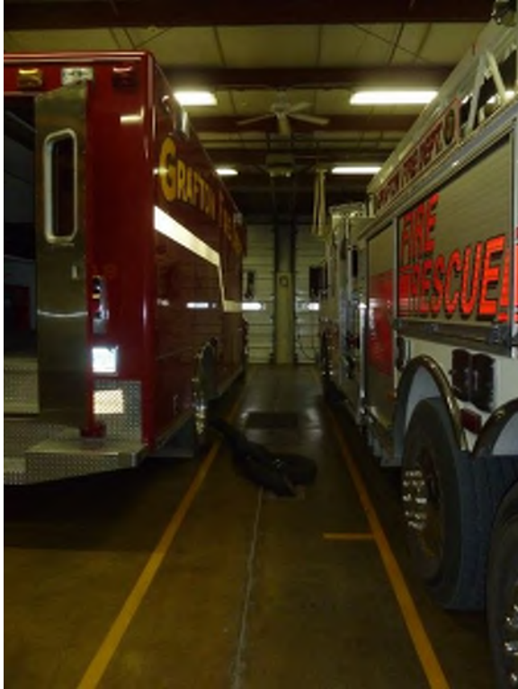
Underslab exhaust hose creates a tripping hazard
