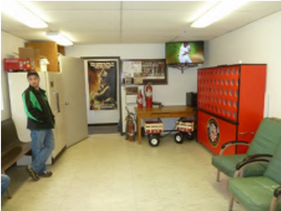
Ceiling tiles exhibit significant sag and are at end of useful service life
