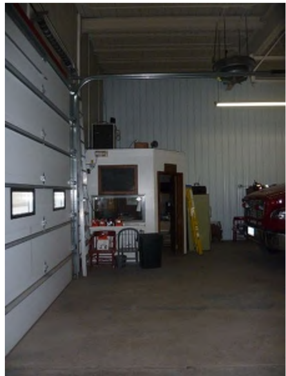
No evidence of code required sand trap/ oil separator from apparatus bay drains
