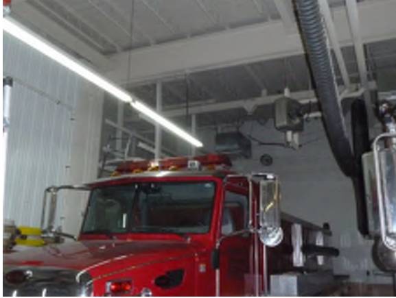
No sprinkler system
