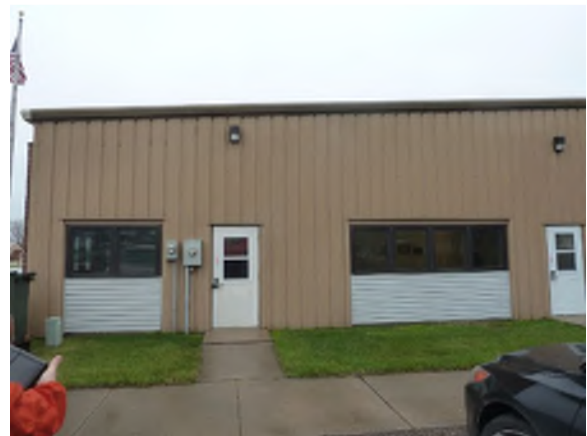
No 5'x5' pad at entry doors
