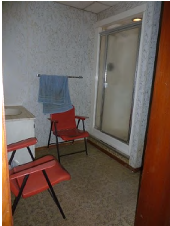
No separate restroom facilities for men and women
