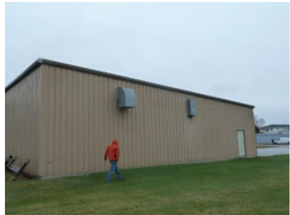
No make-up-air for exhaust system requires exterior doors to be propped open when exhaust is operating
