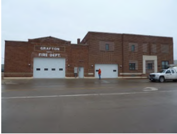
Pedestrian entry into station during a call crosses apparatus response path
