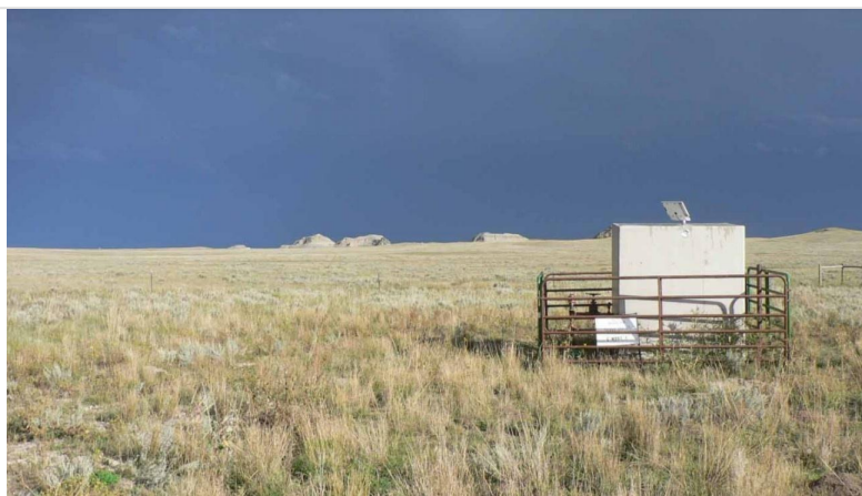
One of the orphaned Spyglass natural-gas wells.
