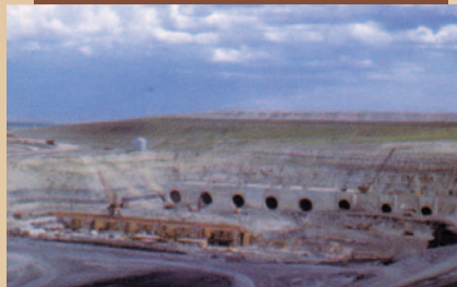
1947: Construction began on Garrison Dam.
