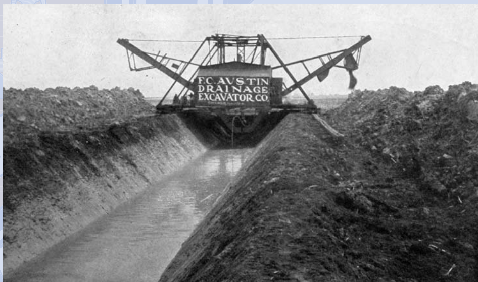
Drainage excavator. (Circa 1905.)
