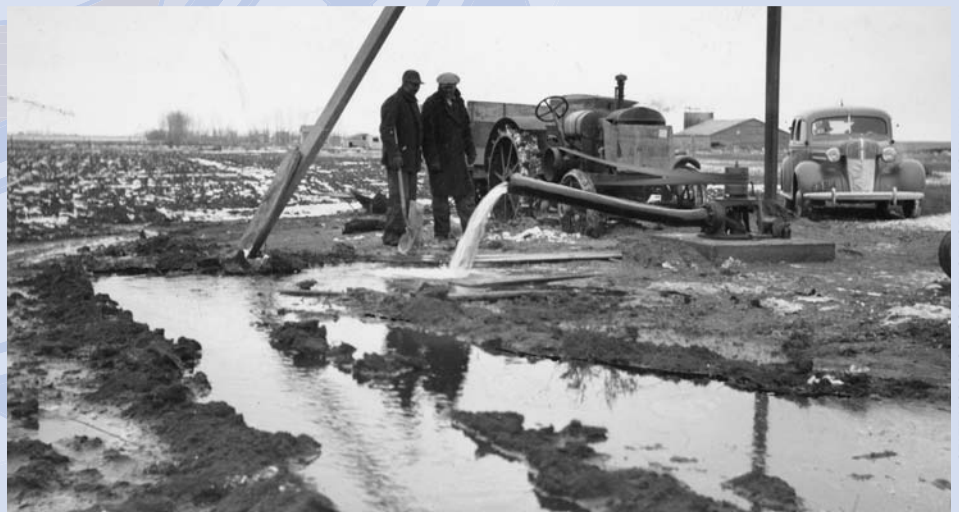
Pumping from a well on the A.L. Maxwell farm, Turtle Lake, ND. First well project developed by the State Water Commission. (1937.)
