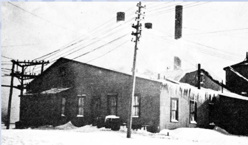
View of the powerhouse at the Wilton Coal Mine, Wilton, ND. (Circa 1916.)
