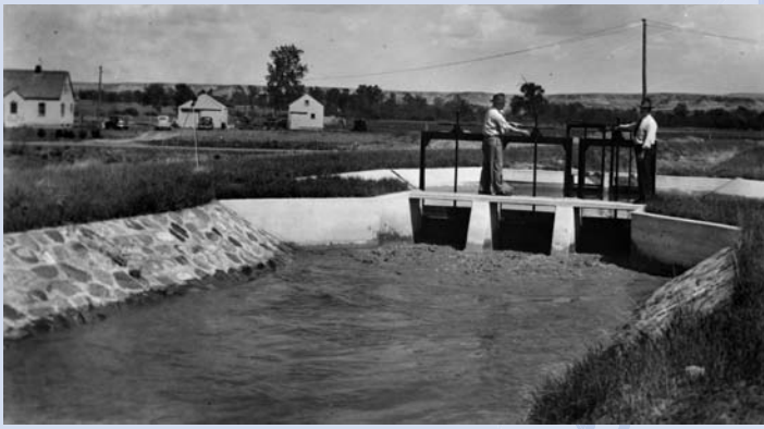
Control gates on main canal of Lewis & Clark Irrigation District, near Williston. (Circa 1945.)
