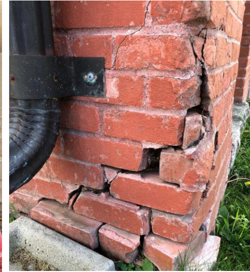
Foundation deterioration and cracking.
