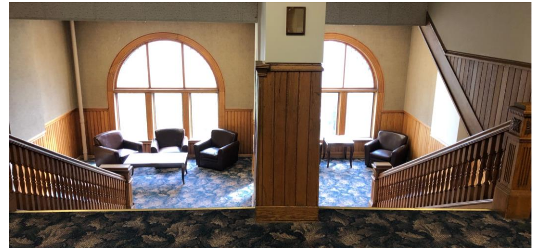
Life safety issues with side-by-side open stairwells.
