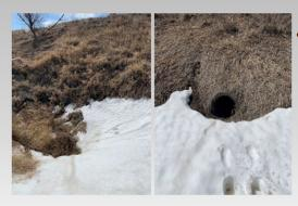
Culverts found in area of major derailment collapsed and plugged not allowing water to drain under roadbed.
