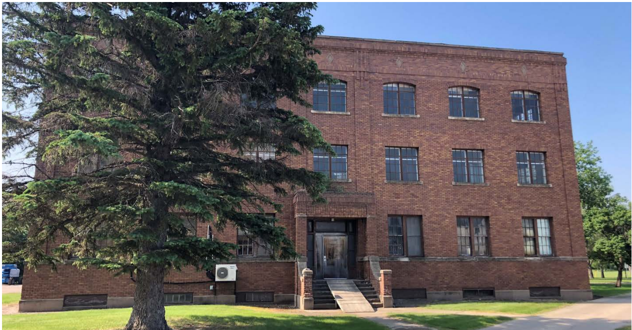
Image 1B: Building 16 East (North Elevation)
