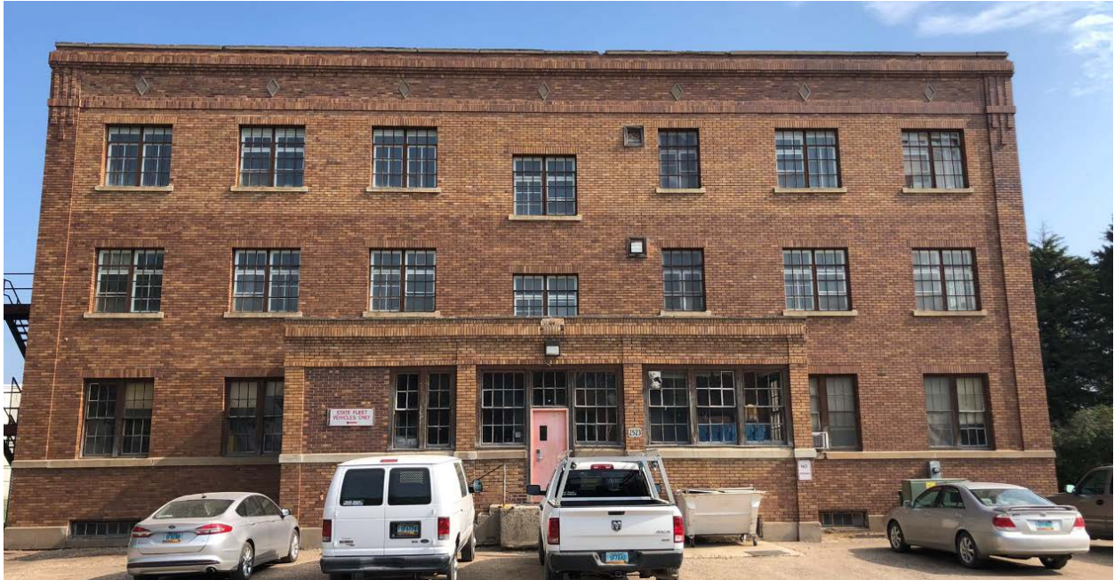
Image 1A: Building 16 East (South Elevation)
