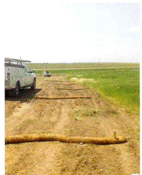
Same site after reclamation
