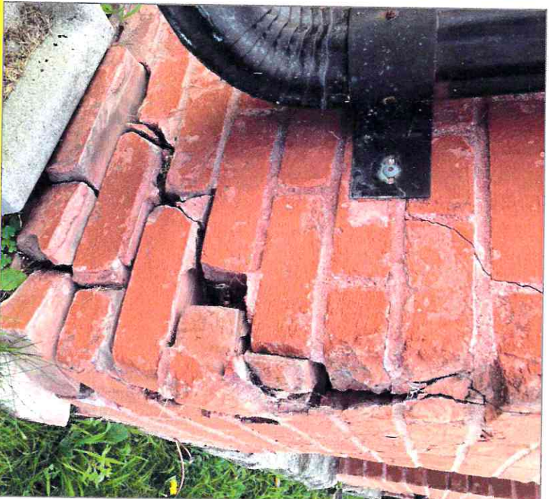
Foundation deterioration and cracking.
