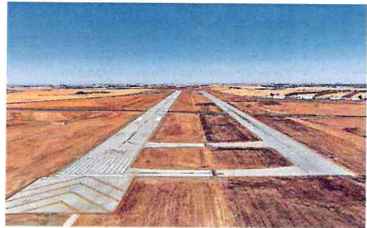
Dickinson Airport Primary Runway Construction (2022)
