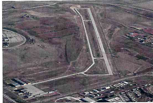
Watford City Airport Runway Reconstruction & Extension (2021)
