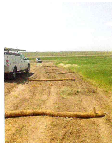
Same site after reclamation
