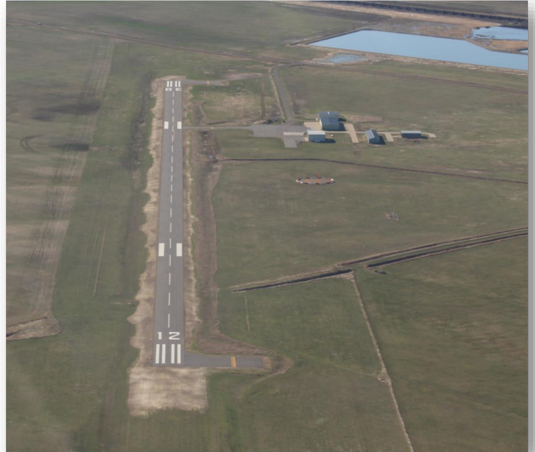
Beach Airport's Completed Runway Rehabilitation
