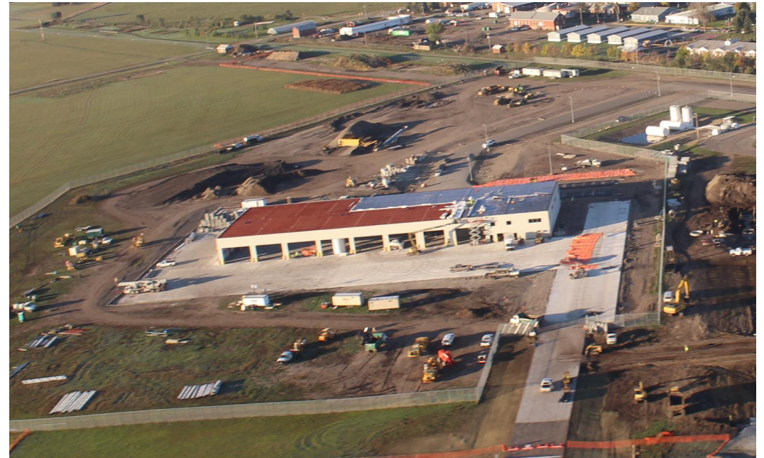
Bismarck Airport's New Snow Removal Equipment Building
