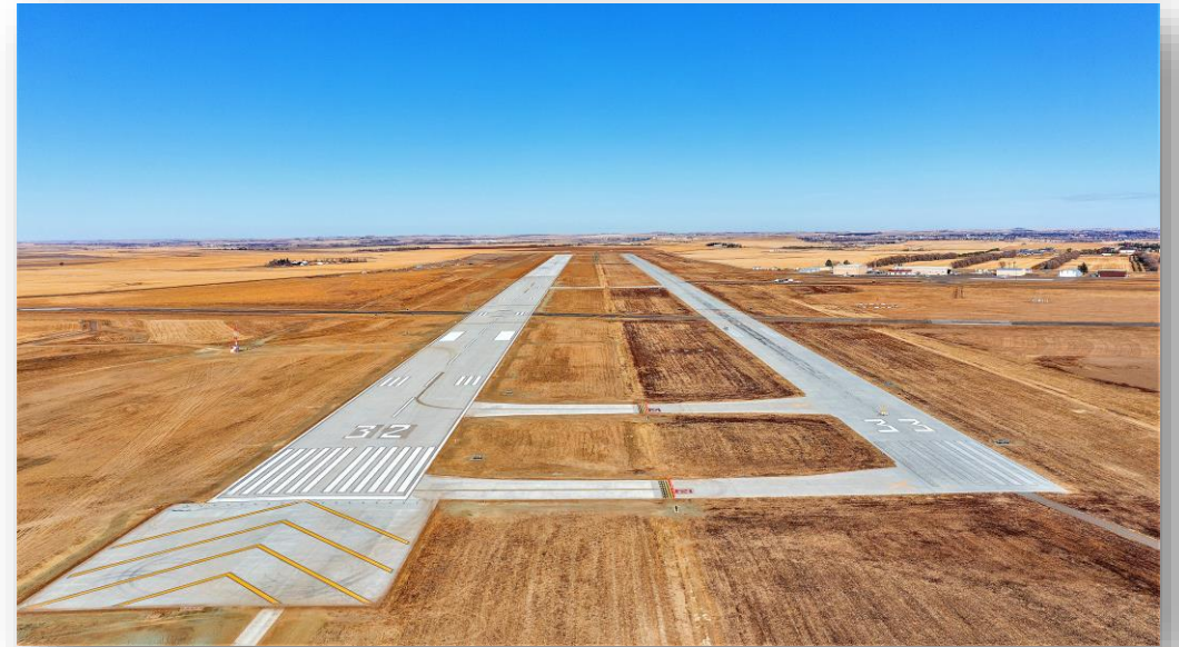
Dickinson's new runway and taxiway opened in November, 2022
