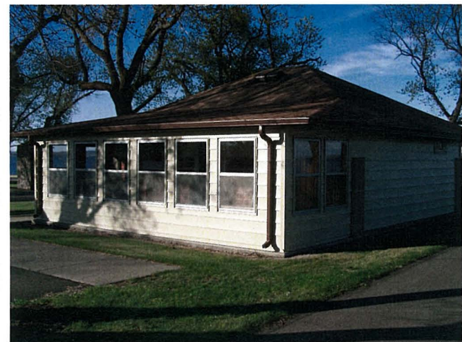
Building #1700, Command Sergeant Major's House
