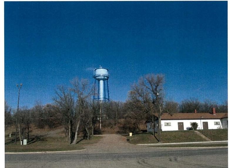
Building #6980, Water Tower
