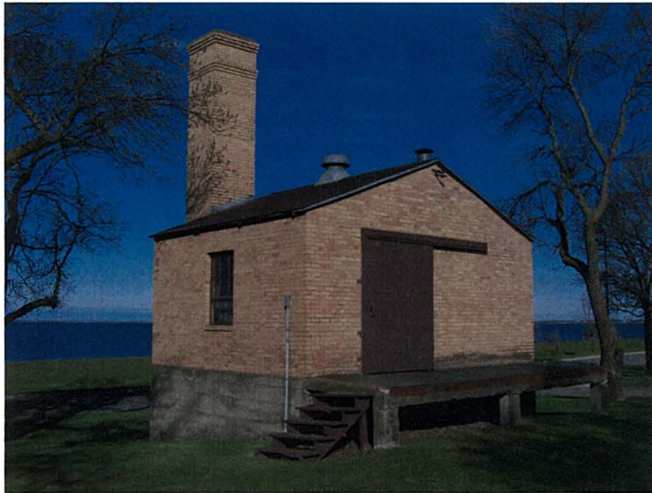
Building #4080, Incinerator building
