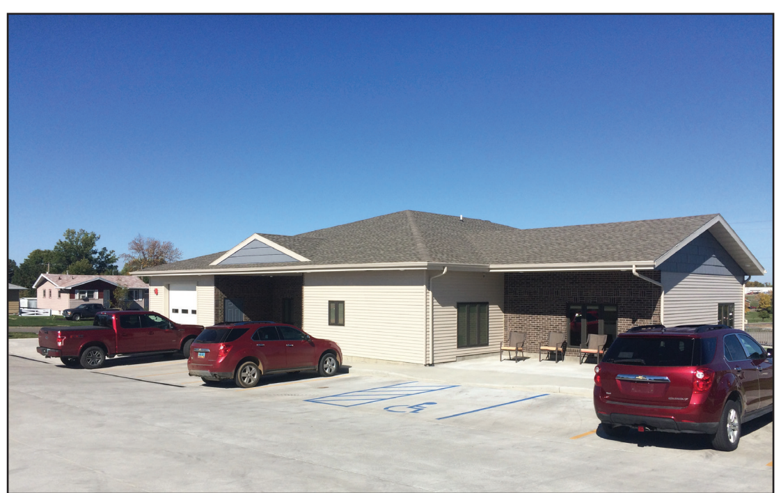
This is one of 10 ICF/IDD group homes - eight of the 10 are in Mandan and two are in Bismarck. Three of the homes are for children and seven are for adults. They also have four homes with up to six beds. HIT, Inc. cares for approximately 115 people and employs 650 people. Pictured is one of HIT, Inc.'s four-bed homes.
