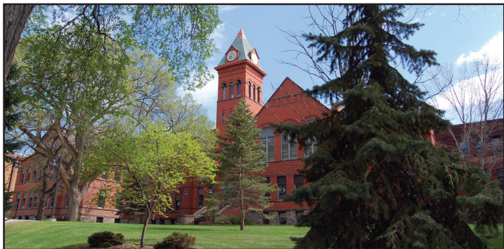
Much has been invested in McFarland Hall over time, but significant deferred maintenance remains.
