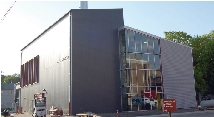
Integrating an activated carbon plant with VCSU's new heat plant will provide a new revenue stream and research opportunities for students and faculty alike.
