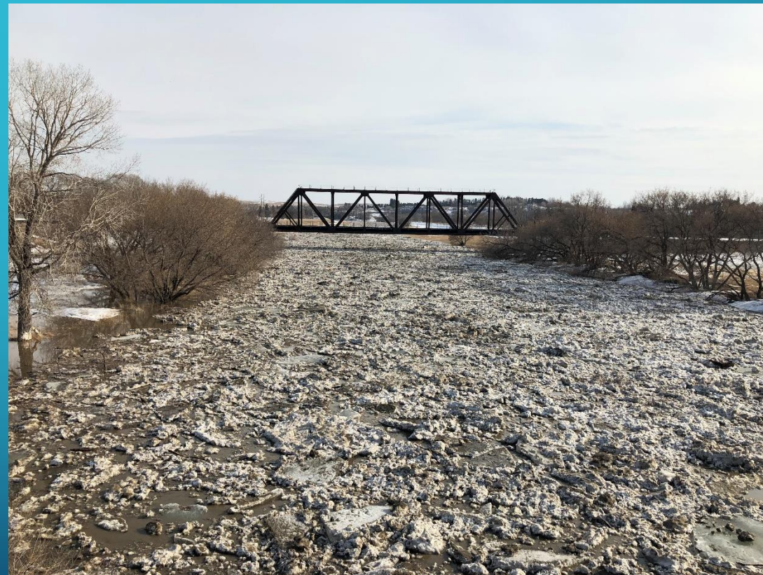
RR Bridge DS of Highway 10 , Mar. 23, 2019
