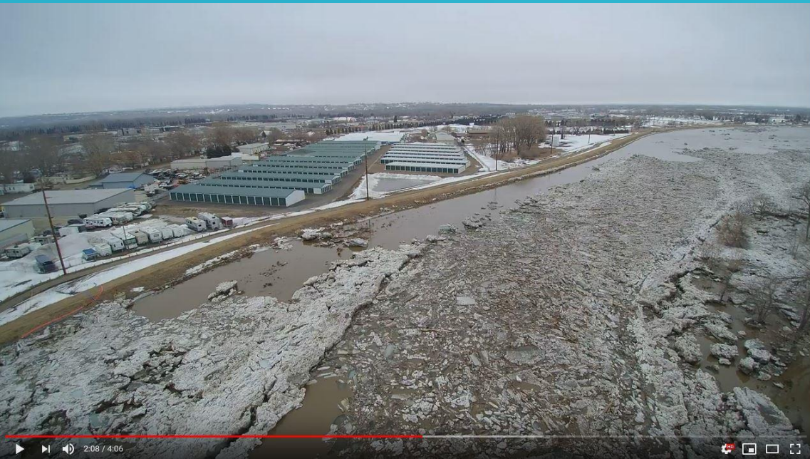
DS of Trolley Bridge, Mar. 26, 2019 – NDSWC Drone Flight
