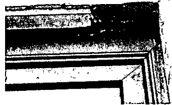
Lintel does not extend full width of opening.
