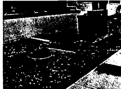
Settlement adjacent to west side of laundry allows ponding.
