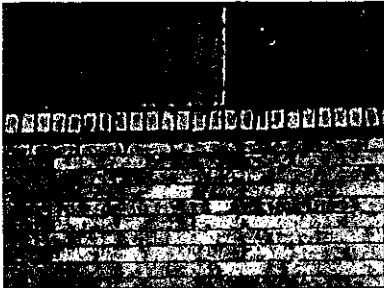
Mortar joints at sill deteriorating.
