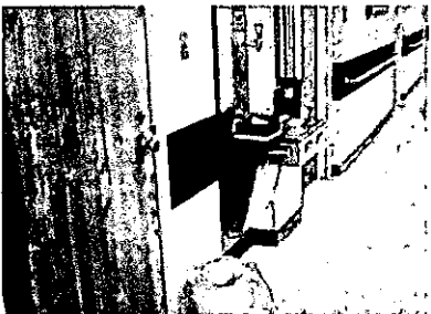
Electric water cooler forms obstacle.
