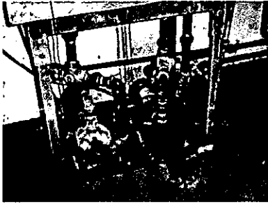
Condensate pumps at boiler #4.
