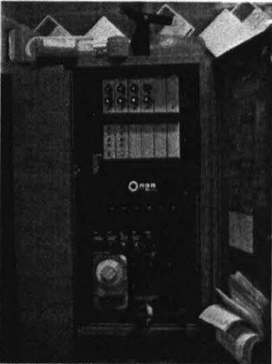
Transfer switch at Onan generator.
