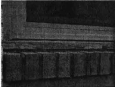
Deterioration of window sill and caulking.
