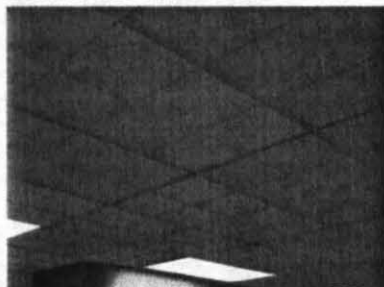
Stained ceiling above serving line.
