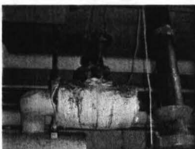
Deteriorating insulation on piping.
