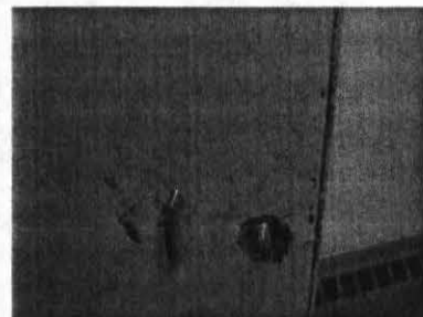
Deteriorating finish on toilet partition.
