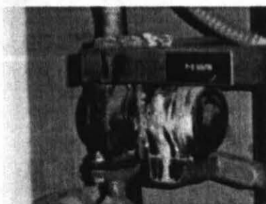
Efflorescence on pump.
