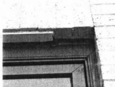
Lintel does not extend full width of opening.
