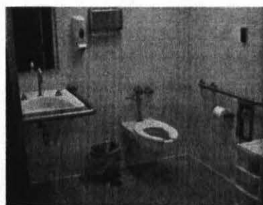
Resident toilet room in 1978 addition; note lack of rear grab bar.
