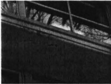
Concrete sun shade spalling.
