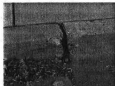
Damaged concrete curb.
