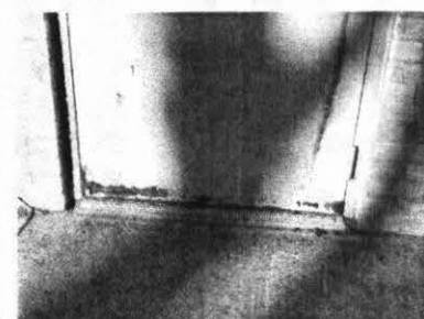
Deteriorating finish and rusting door.
