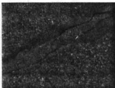
Crack in asphalt paving. Note ravelling.
