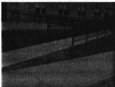
Lack of handrail extensions at ramp.
