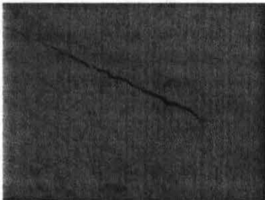
Crack in surface of roof repair.
