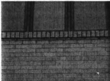
Mortar joints at sill deteriorating.
