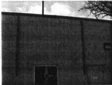
Angles used to secure tie rods through building.
