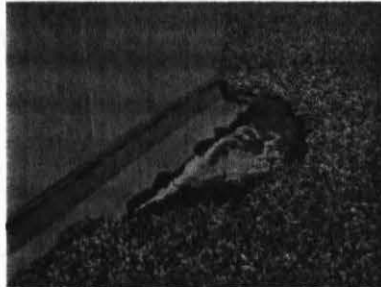
Aggregate surfacing shifting.
