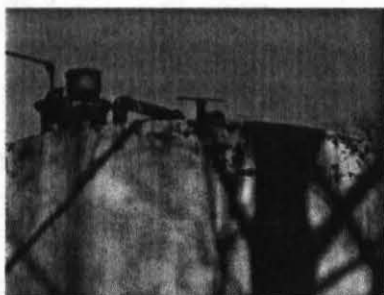
Deteriorating finish on fuel storage tanks.
