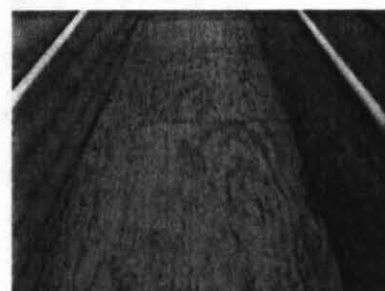
Finish on ramp at Gazebo deteriorating.
