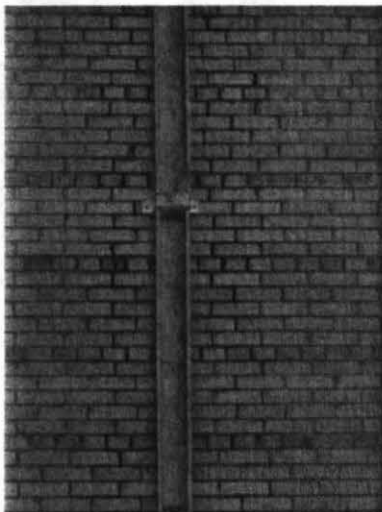
Mortar joints behind downspout deteriorating.
