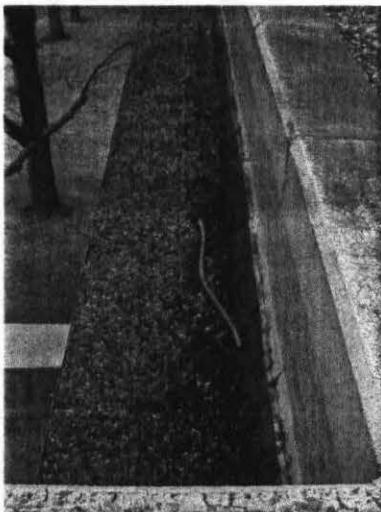
Built-up roof on sun shade.
