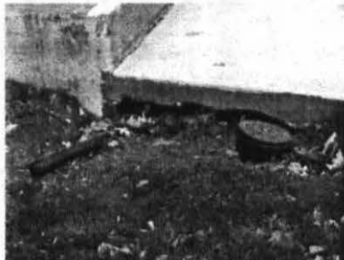
Erosion under sidewalk at north end of building.
