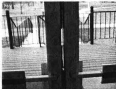
Lack of weatherstripping between door leaves.
