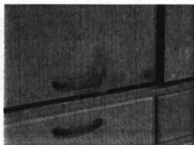
Deteriorating cabinets in original portion of building.
