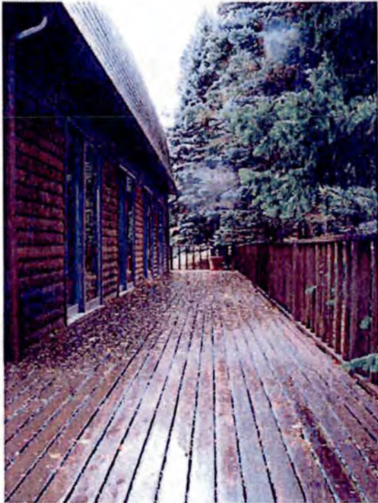
View of Deck Surrounding Lodge and Barn
