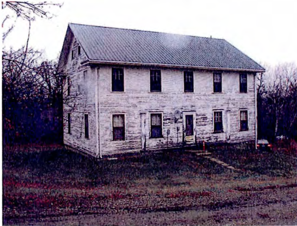
Front View of Dorm Building – Looking Northerly
