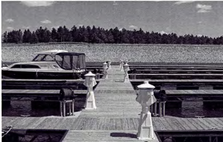
FSSP docks electrical
