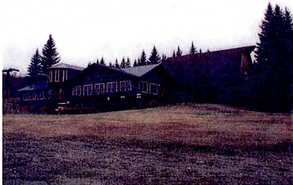
View of Lodge Building and Barn – Looking Southwesterly
