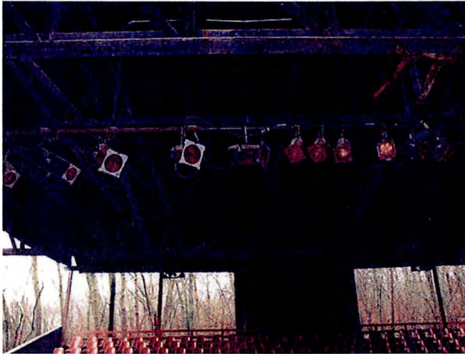
Amphitheater Lighting and Ceiling
