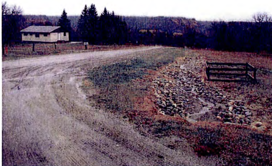
County Road 55 – Looking Easterly
