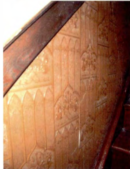
Detail of wall panels at stairway
