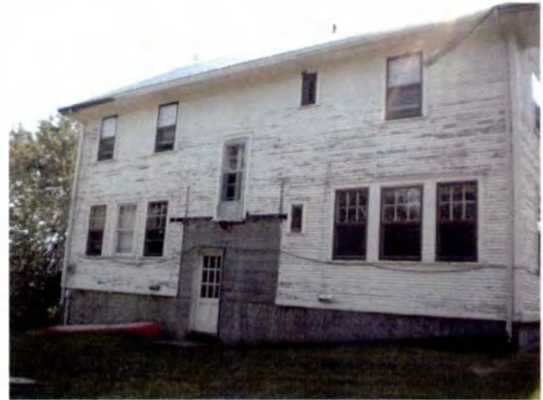
Back of Dorm – back entry structure removed
