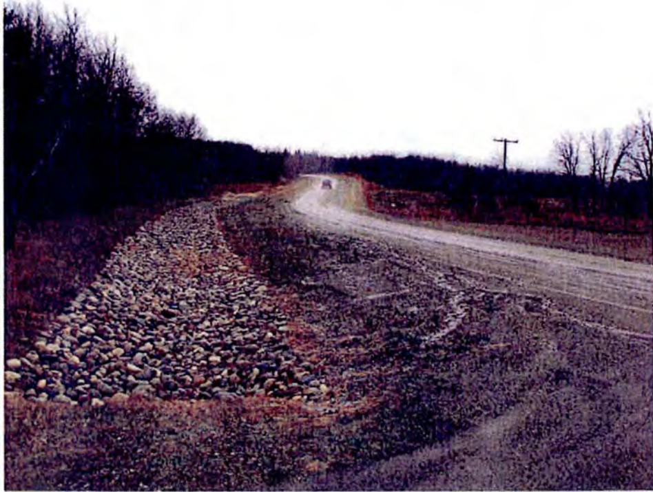
County Road 55 – Looking West
