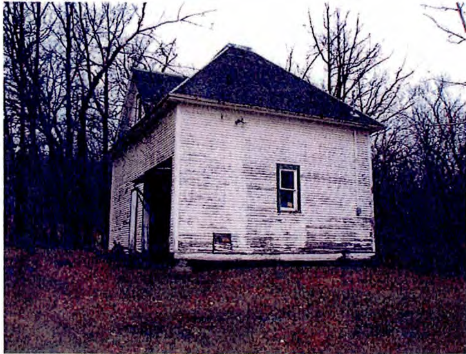
Carriage House (To be removed by current property owners)
