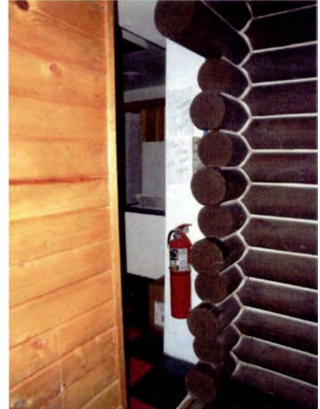
Detail of the Log structure
