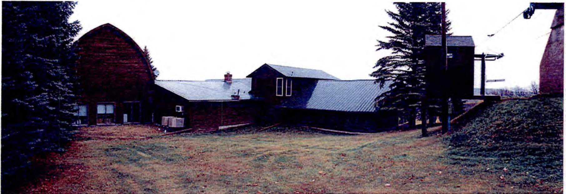
Rear of Barn and Addition to Lodge Building – Looking Northeasterly
