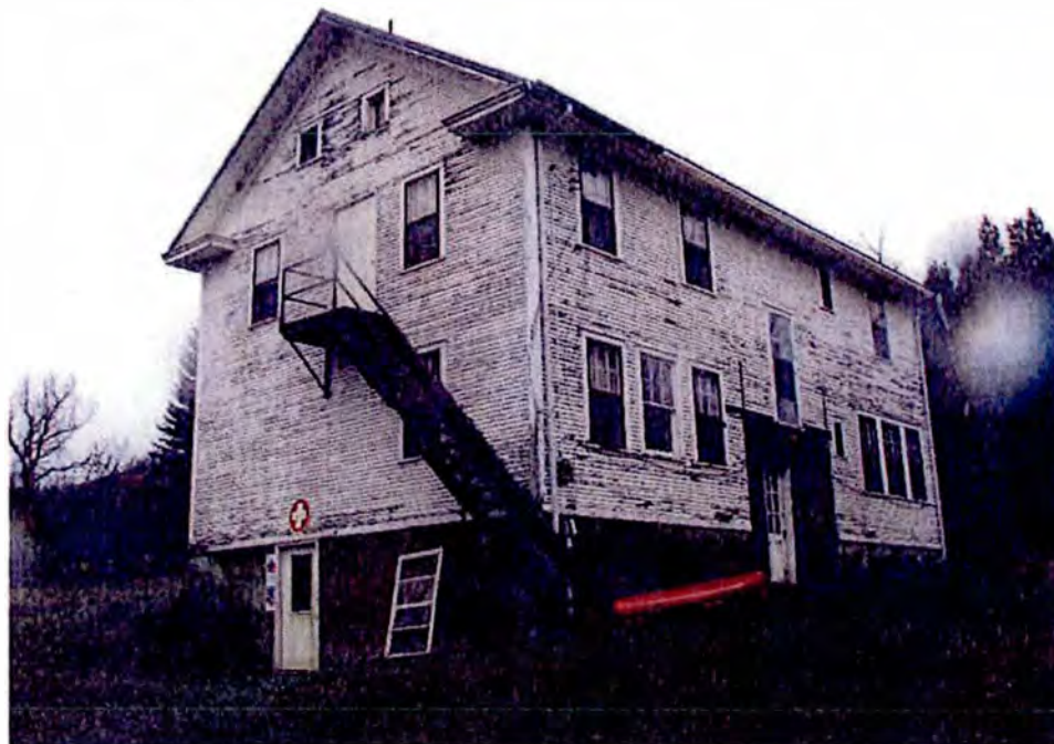
Rear View of Dorm Building – Looking Southwesterly
