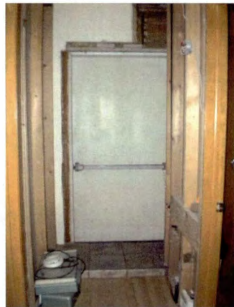
Second floor – fire escape door
