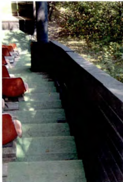
Side aisle with half wall
