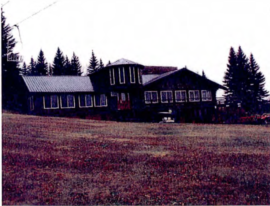
Front View of Lodge Building – Looking West
