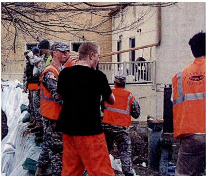
As the Sheyenne River winds through our communities, areas on both sides of the river need protection. In Valley City, dike work covered nearly seven miles. During the last flood, a combination of sandbag, clay dikes, hesco barriers and aqua dams were placed.
