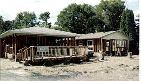
Many homes in Minot were so badly damaged by floodwaters, they had to be stripped down to the studs.
