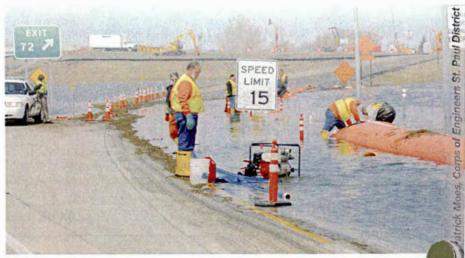
The exit to Harwood from I-29 was closed due to water on the road. At the height of the 2011 flood, the Fargo-Moorhead area and rural Cass County experienced 100 miles of closed roads, many washed out roads and culverts, and significant damage to area bridges.
