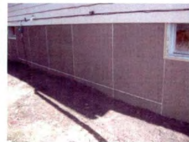
Installation of foundation paneling
