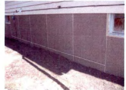
Installation of foundation paneling
