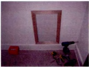
Quality finish work on the entrance to this crawl space.
