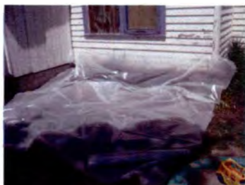
Ensuring ground is protected from lead paint chips
