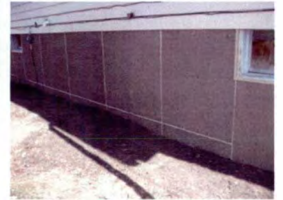
Installation of foundation paneling
