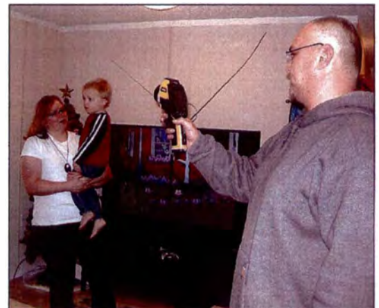
Bill Swartwout with Community Action Partnership holds an infrared camera to check for air leaks in a FEMA home as resident Jerusha Schiessl and son Austin watch in the background.
