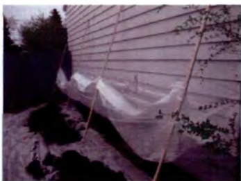
Ensuring ground is protected from lead paint chips
