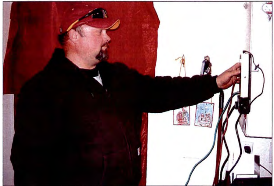
Bill Dunn with Community Action Partnership, standing in front of a door with a blower fan, sets up to conduct a test to check for tightness of a FEMA home in southeast Minot Tuesday.
