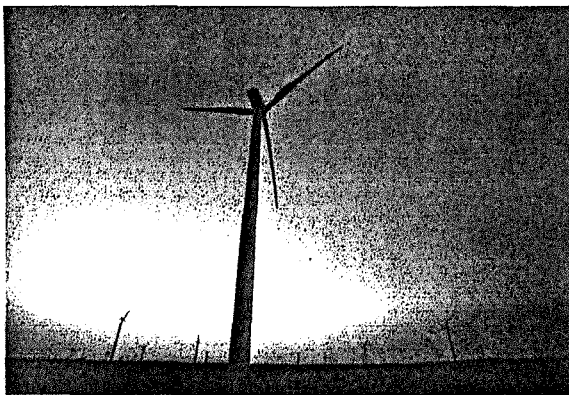
Picture: 1.5 mW GE Turbine.
