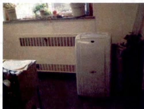
Figure 1 - Portable Air Conditioner and Steam Radiation
