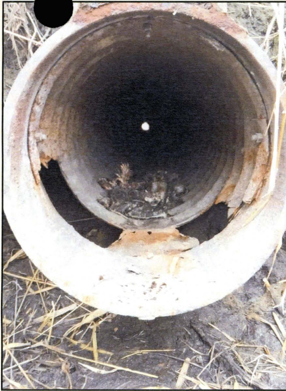
Rusted out 15" Culvert
