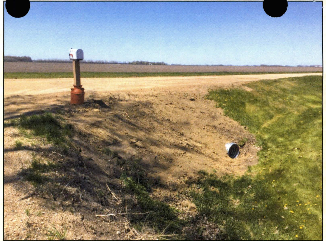
18" Replacement Culvert Installed
