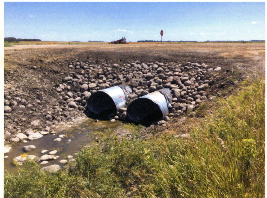
Drain 31 Culvert Replacement Complete Downstream End
