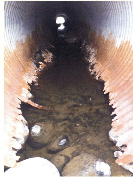
Drain 31 Culvert Damage
