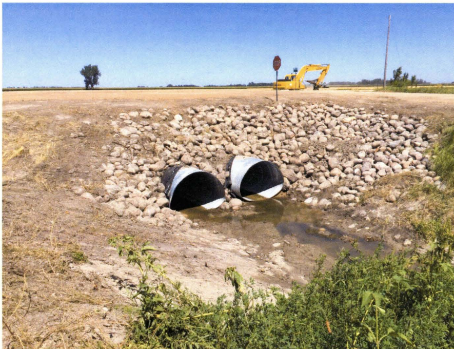
Drain 31 Culvert Replacement Complete Upstream End
