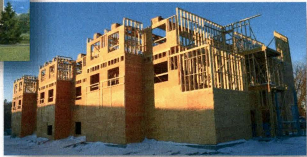
Construction Progress, January 2019
