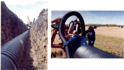
Agassiz Drain Tile
