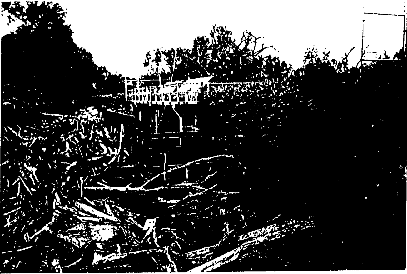
Logjam at trashrack on Eaton Dam
