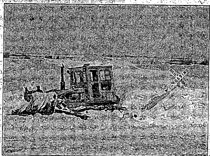
Working to clear one of the crossings.
