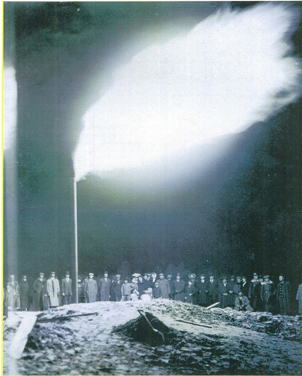
Gas flair from sandstone at a depth of 250 feet near Mohall in the early 1920s.
