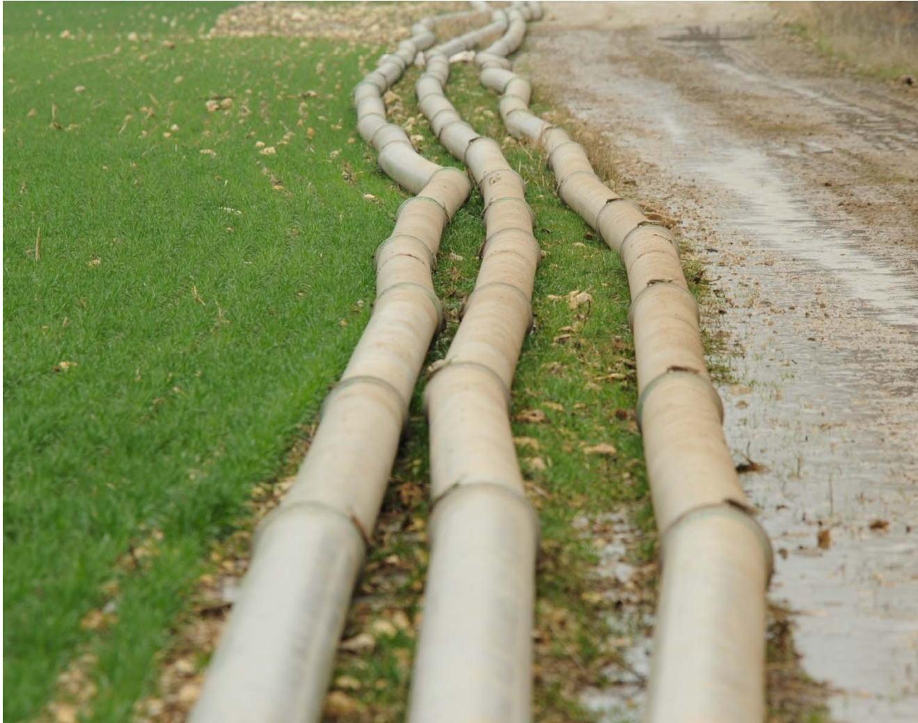
Temporary lines take water to well site
