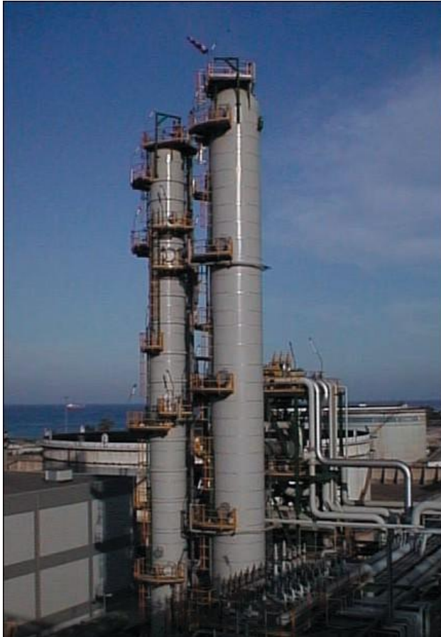
Industrial-Scale Monoethanolamine (MEA) CO 2 Scrubber
