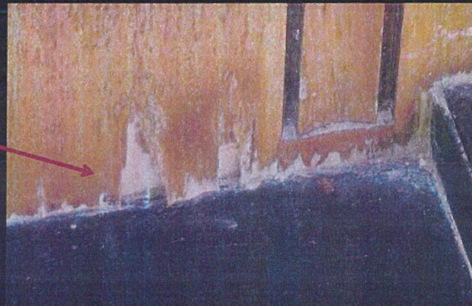
Window Sill @ West End of Legislative Wing showing Cracked Marble and Delaminated Wood Sill/Jamb
