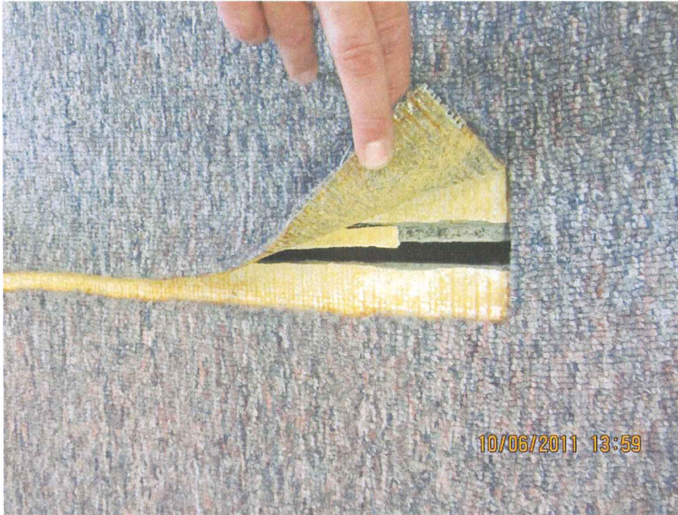
Photo #3: Separation of the slab-on-grade construction joint at the interior steel column locations.
