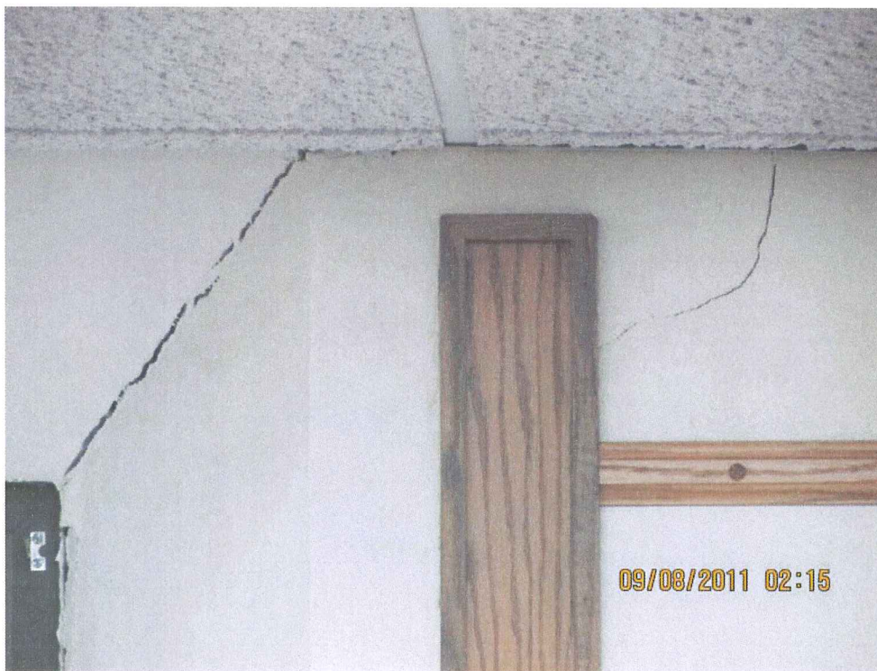
Photo #12: Cracking of interior wall finishes on west side of library.
