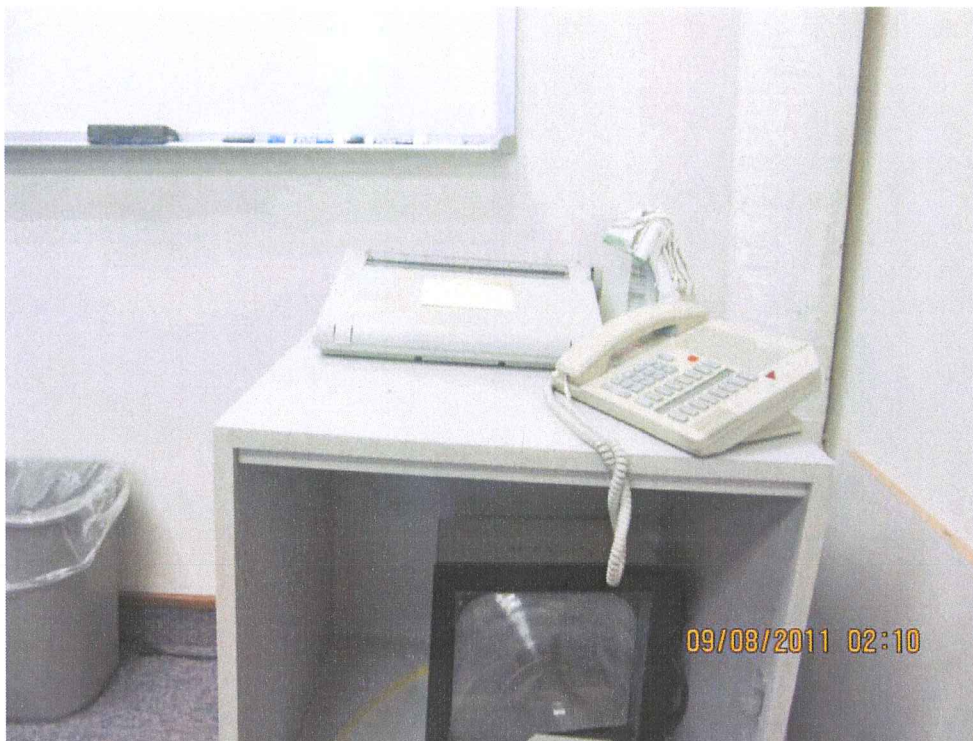
Photo #13: Leaning counter due to sloping floor in CCTV Room on west side of building.
