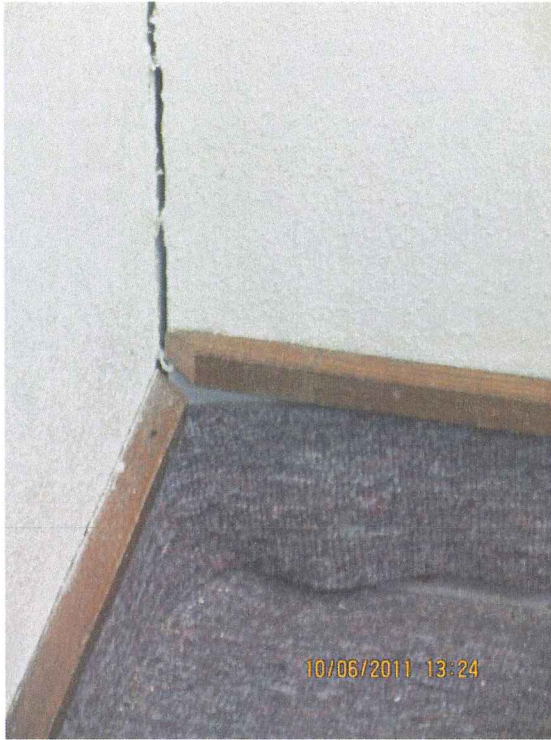
Photo #1: Separation of interior wall and finishes from the west exterior wall (base of wall).
