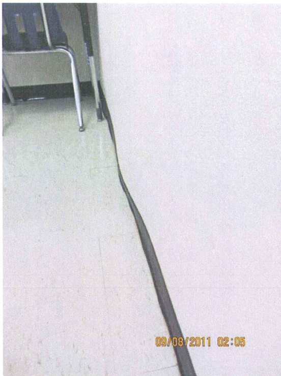
Photo #7: Buckling of wall finishes at classrooms on north exterior wall.
