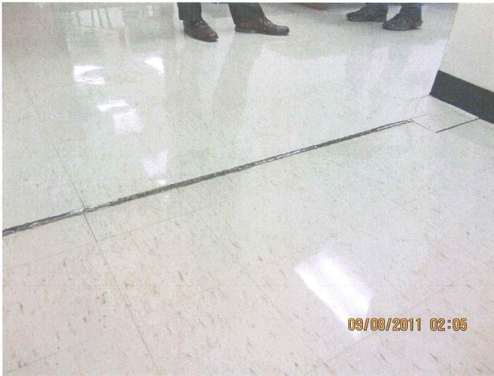
Photo #11: Movement and vertical separation in slab joint in classroom corridor on north side of the building.
