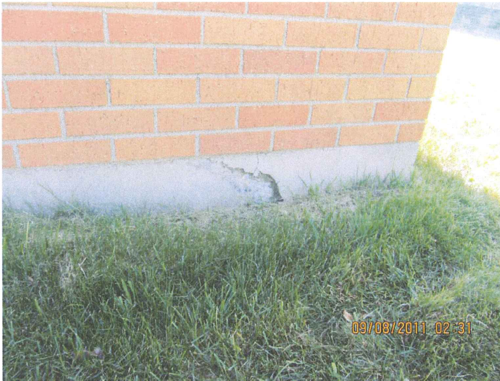
Photo #15: Signs of distress in the foundation wall on the west side of the building.
