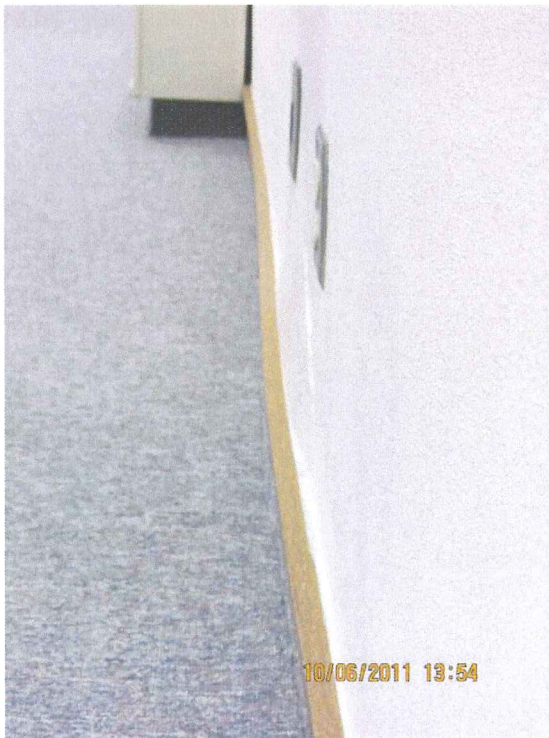
Photo #4: Buckling of wall finishes at west exterior wall.
