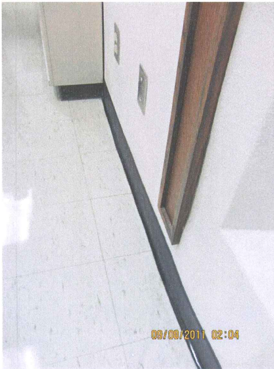
Photo #10: Buckling of floor and wall finishes on north exterior wall of classroom.
