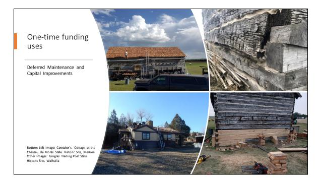
At Gingras Trading Post, the wall of the trading post was stabilized and the roof reshingled.
