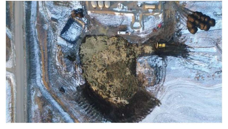
Photo #8 Placing gypsum and straw amended soil over capillary break.
