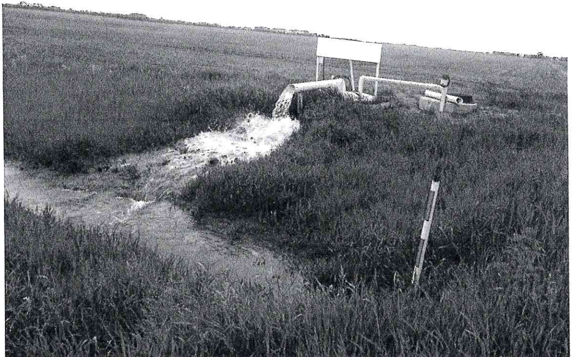
Drainage pump station discharge mixes with surface runoff.
