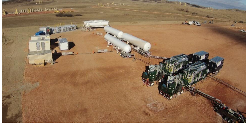
Figure 5: 2 MMCFD of installed GTUIT flare capture equipment along with well site LNG production
