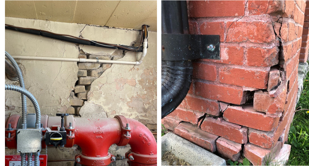
Foundation deterioration and cracking.
