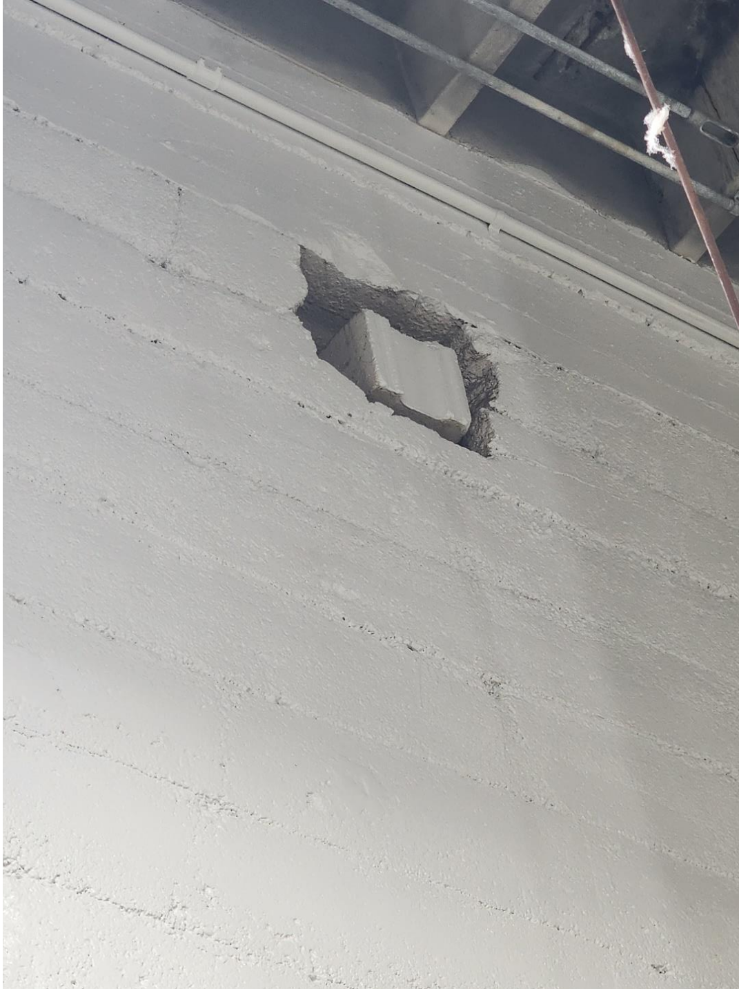
Wall penetrations infilled with non-standard construction methods. Non-rated ceiling assembly as required by building code. Location of water and pest infiltration. (Photo: 20240411_135834)
