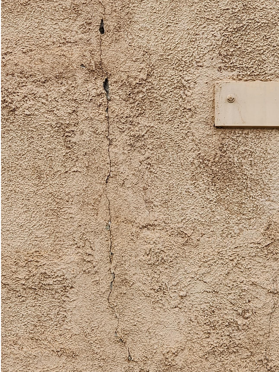
Exterior EIFS in poor condition. Extensive cracking and evidence of water infiltration causing material failure. (Photo: 20240216_143856)
