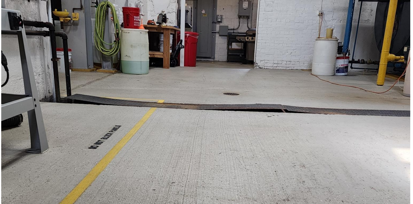
Bent trench drain covers within interior floor slab – potential tripping hazards. (Photo: 20240411_141837)
