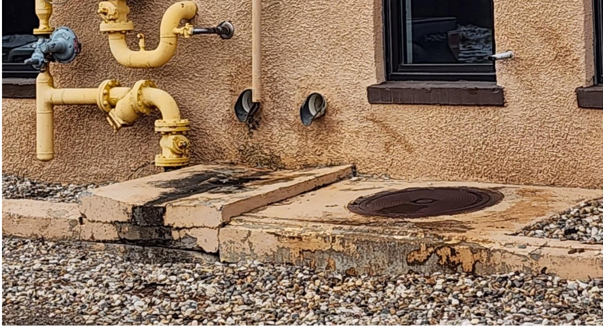
Exterior drainage along wall and foundation in poor condition. Evidence of water infiltration. (Photo: 20240216_1440009)
