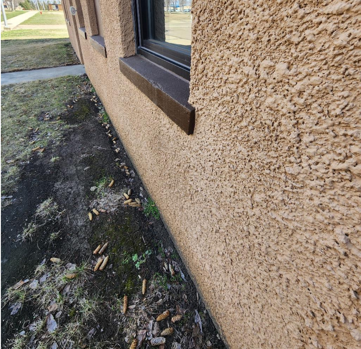
Exterior drainage along the wall and foundation in poor condition. Evidence of water sitting along the foundation wall. (Photo: 20240411_145949)
