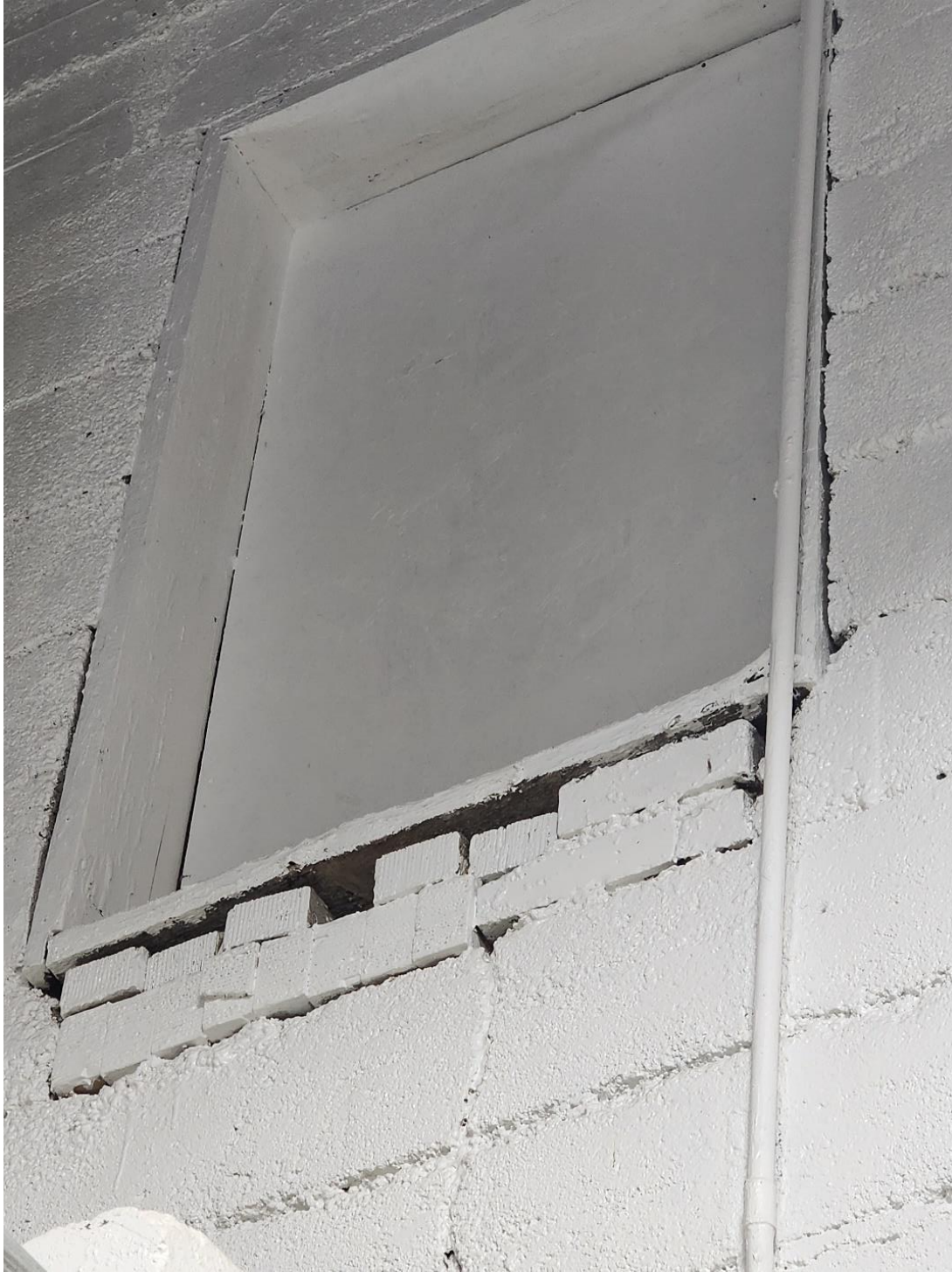
Window jambs and sills in poor condition and non-standard construction methods. Location of water and pest infiltration. (Photo: 20240411_135835)
