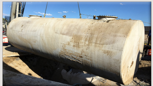
Removing an underground storage tank
