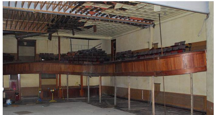
Before a new roof was installed in the 1990's, water damaged and warped the auditorium balcony. The balcony originally was hung from the roof by metal rods, but new steel supports extending from the basement to the third level will need to be installed before the restoration of the balcony can be completed.
