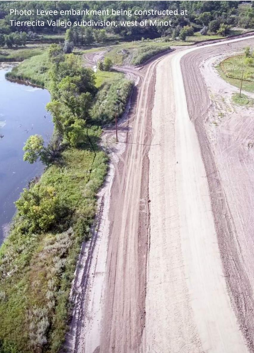
Photo: Levee embankment being constructed at Tierrecita Vallejo subdivision, west of Minot
