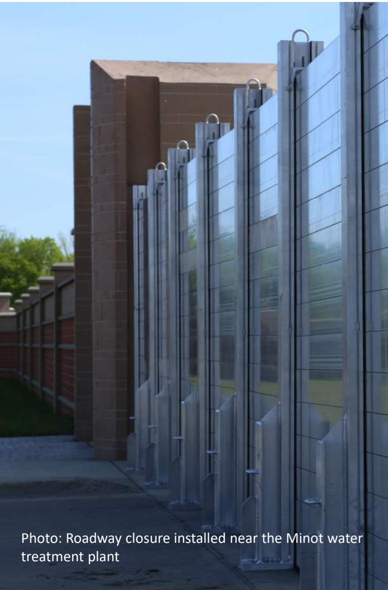
Photo: Roadway closure installed near the Minot water treatment plant
