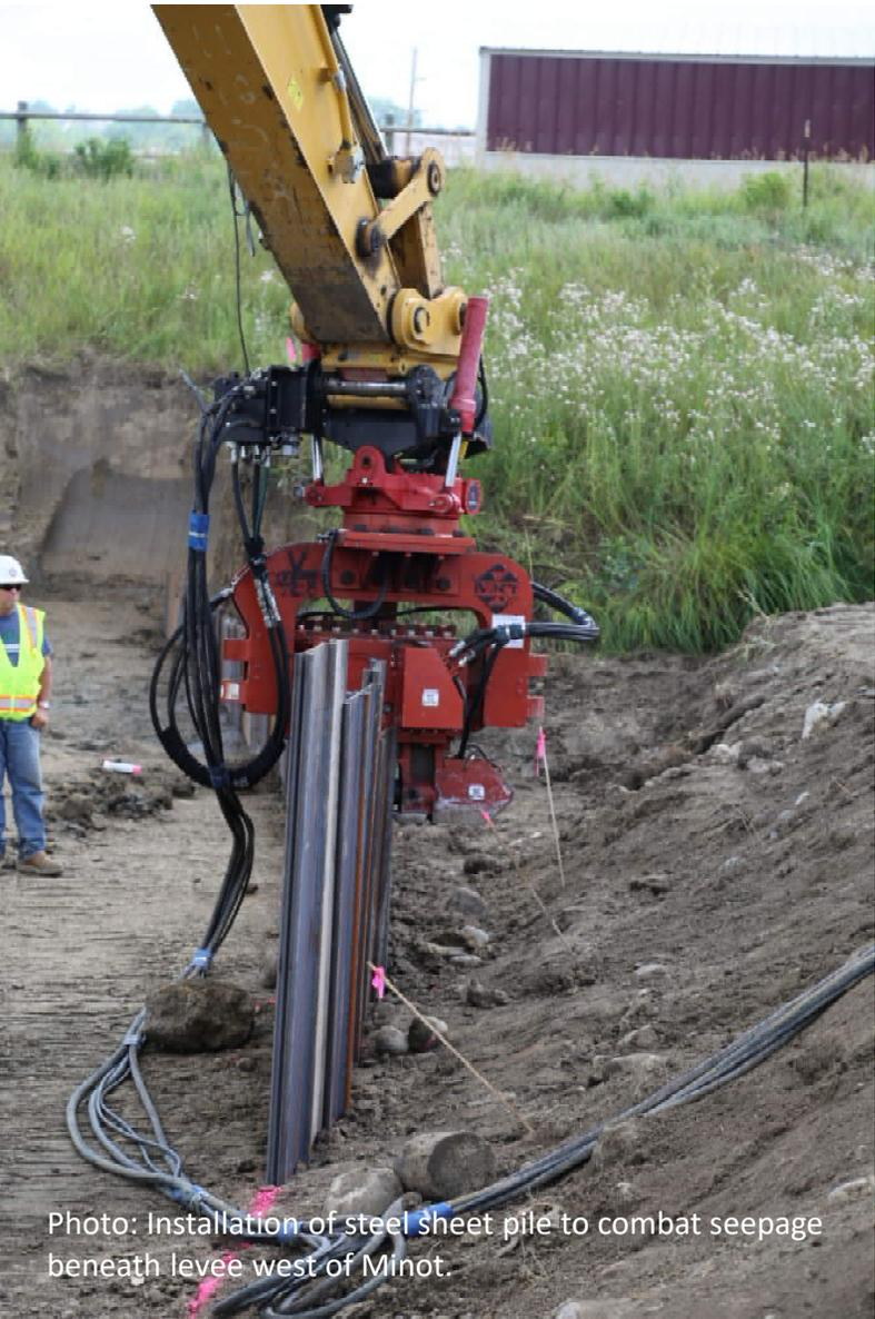
Photo: Installation of steel sheet pile to combat seepage beneath levee west of Minot.
